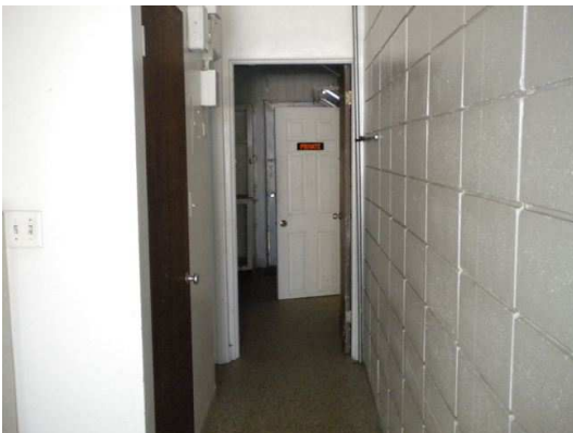
EAST SIDE HALLWAY
